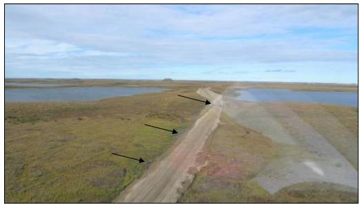
Figure 14 Multiple areas of water ponded against the Source 177 road.
