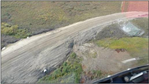
Figure 17 Another area of embankment material slumping and flowing across the tundra.
