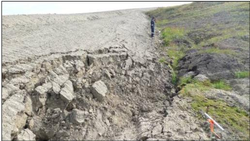
Figure 16 Slumping of Source 177 road embankment material.
