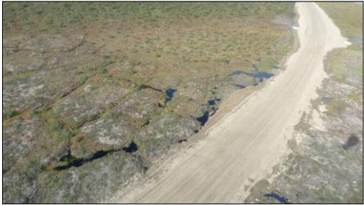
Figure 15 Ponding of water and enlargement of ice-wedge troughs next to the Source 177 road.
