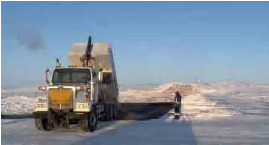
Photo 5.9-3 Example of geotextile placement and end dumping method of construction. (Tuktoyaktuk to Source 177 Access Road, 2009)
